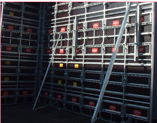
Push-pull prop and push-pull prop "G"
